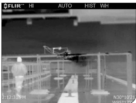
Ammonia (NH 3 ) gas escaping from pipes
